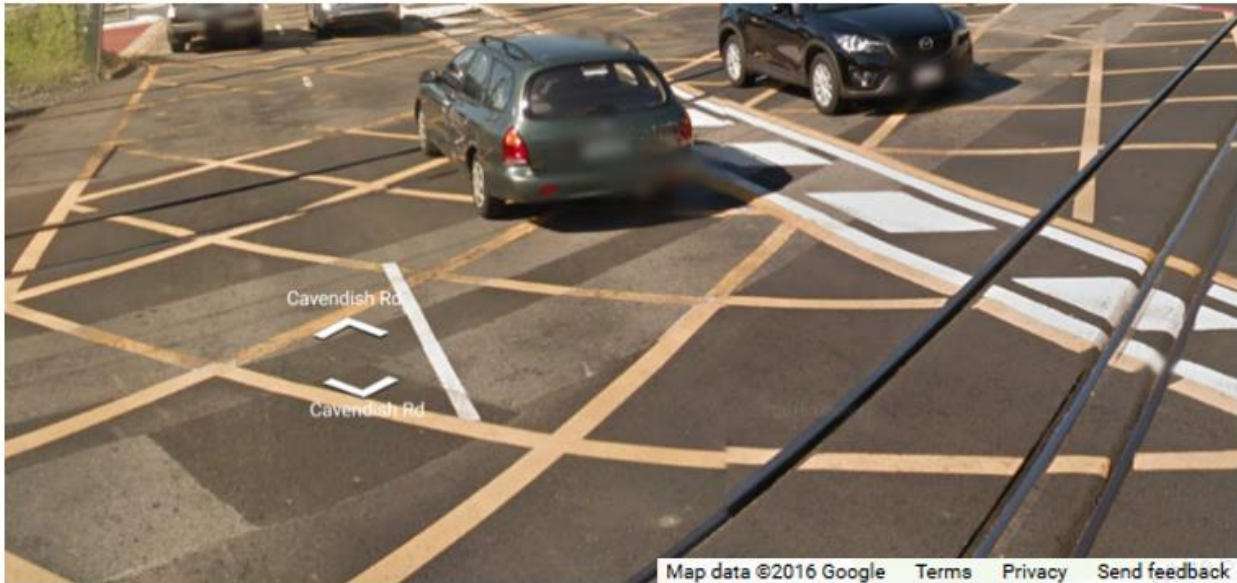
Figure 4.72: Railway crossing hazards
