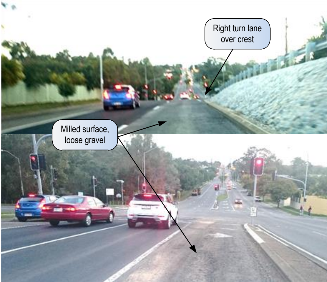
Figure 4.59: Road works, milled surface with gravel spill from asphalt works in through lane and right turn lane
