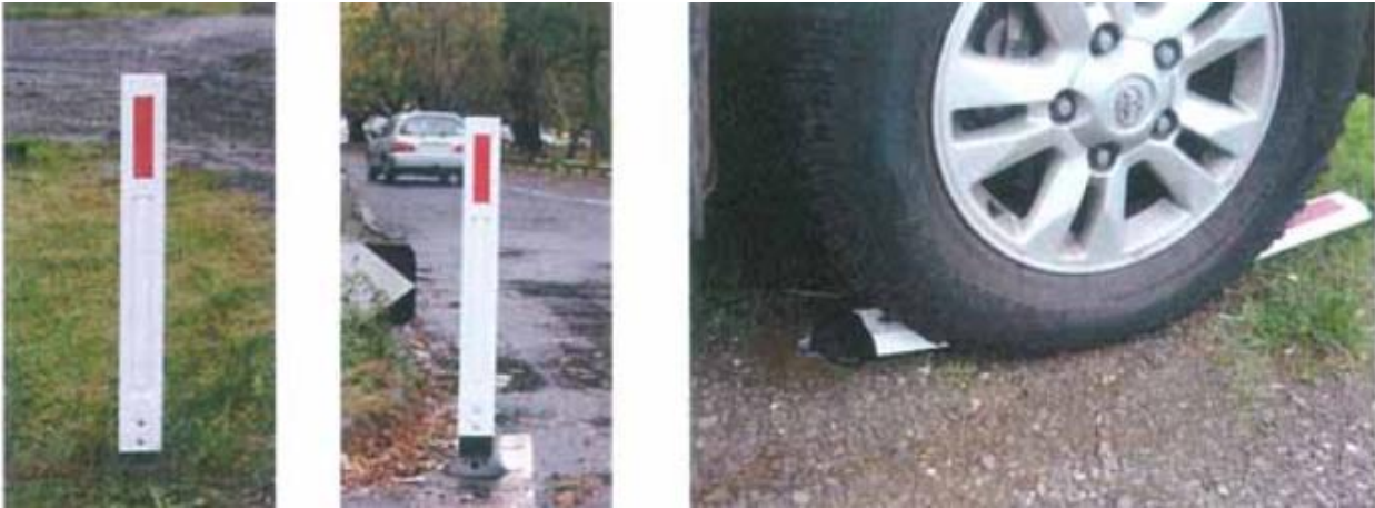
Figure 5.13: Flexible guide posts
