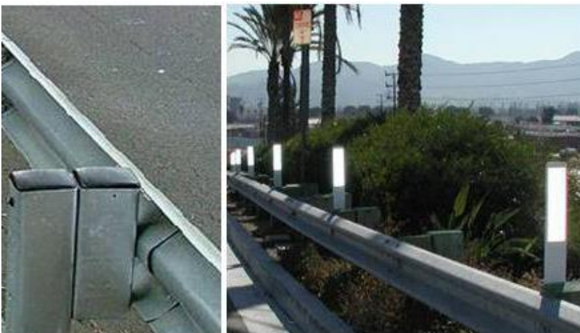
Figure 5.15: Guardrail post caps and flexible delineators
