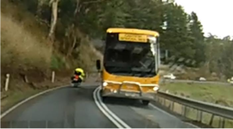
Figure 4.24: Narrow lane and shoulder width
