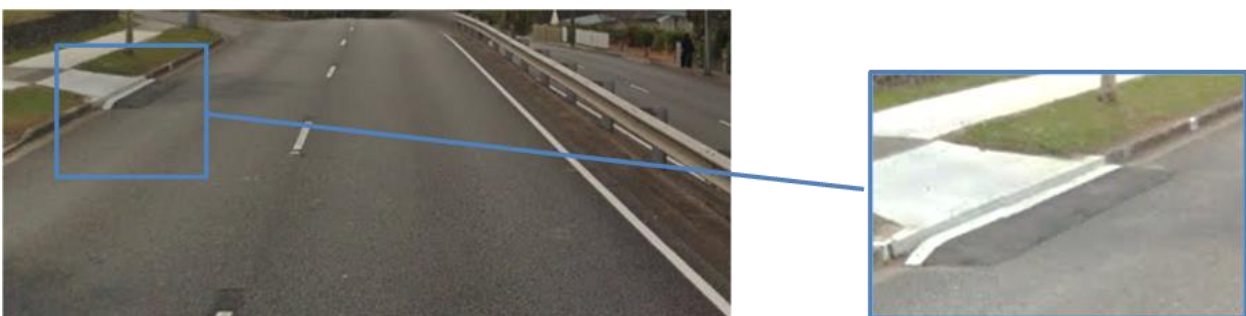
Figure 4.64: Driveway kerbing in shoulder
