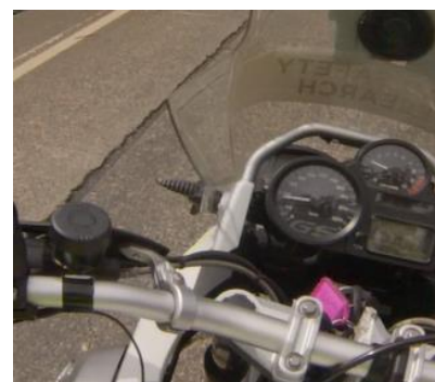
Longitudinal cracking on concrete slabs
