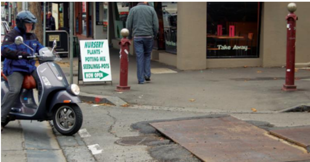
Figure 4.60: Steel plates over trenches
