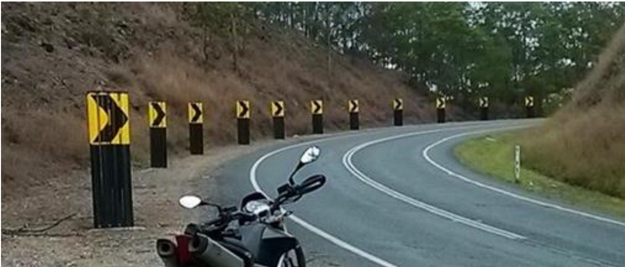
Figure 5.9: Flexible chevron alignment markers
