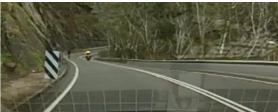
Figure 4.31: Hazard sign on drainage ditch
