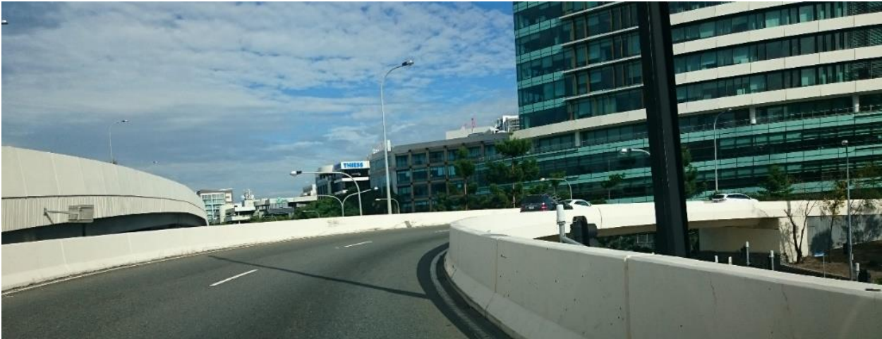
Figure 4.17: Restricted sight lines – right hand curve on interchange ramp
