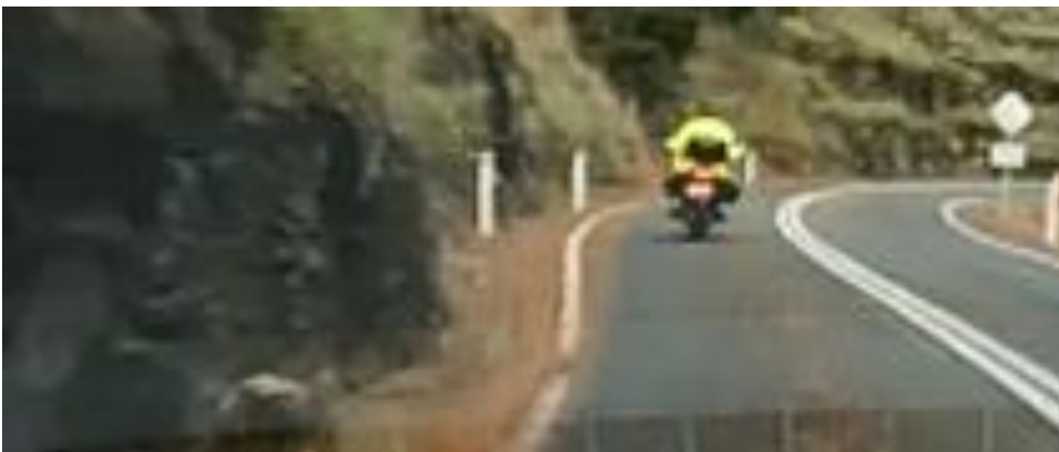
Figure 4.122: Aggressive rock face on cutting
