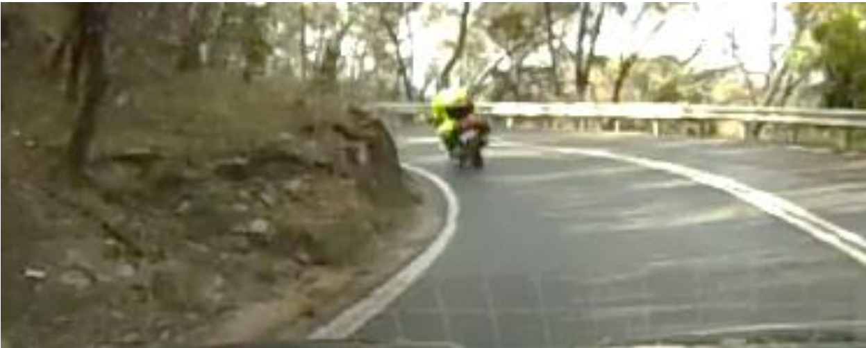
Figure 4.16: Restricted horizontal sight line on sharp curve with narrow sealed shoulders and adjacent aggressive rock face
