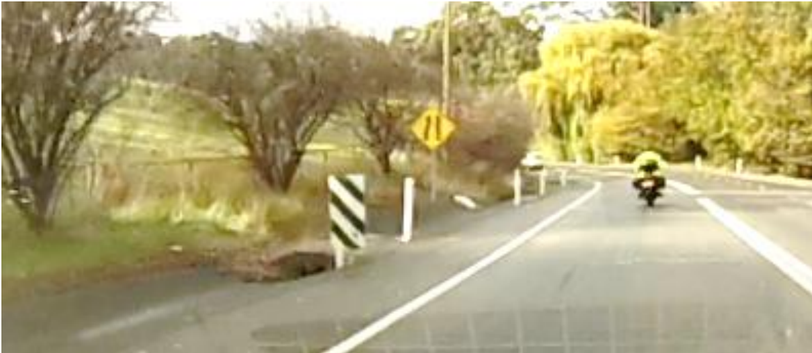
Figure 4.29: Hazard sign on perpendicular culvert
