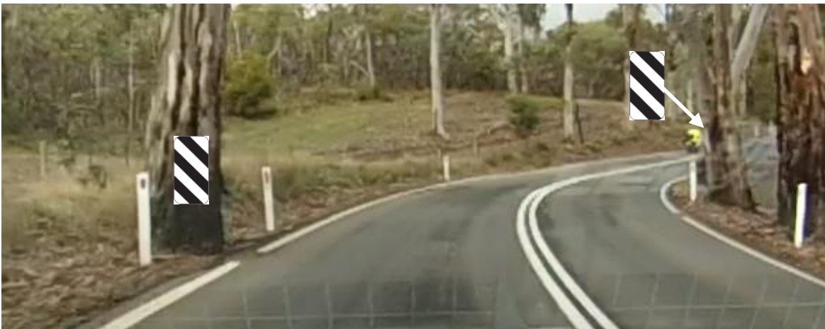
Figure 4.30: Hazard sign on trees in shoulder
