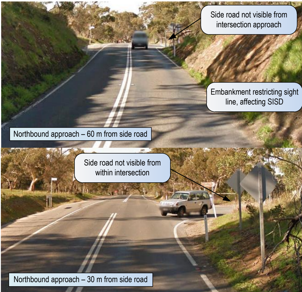
Figure 4.79: Rural – restricted safe intersection sight distance and visibility to side road from approach
