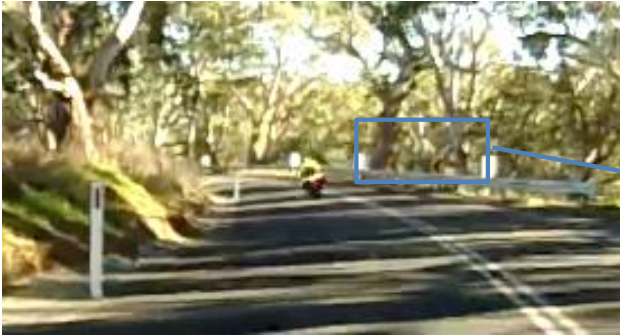
Figure 4.42: CAMs blending into background and hidden by guard rail
