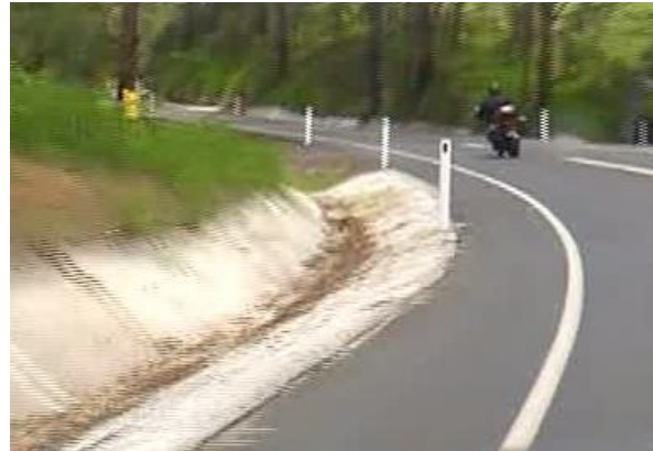
Traversable drainage treatment
