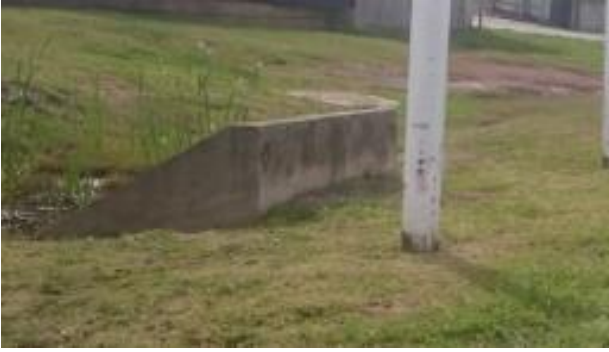
Figure 4.117: Raised culvert wing and headwall
