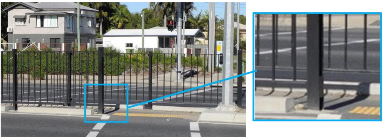
Figure 4.107: Non-frangible pedestrian fencing
