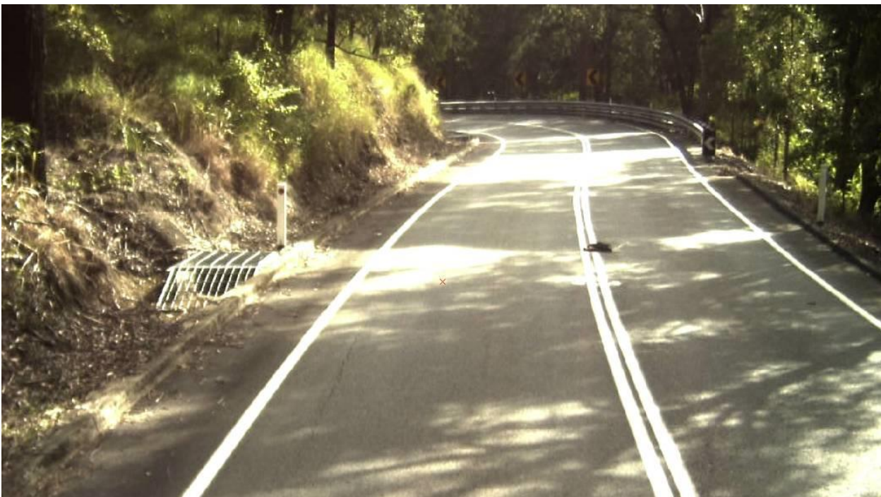
Figure 5.10: Traversable grate over perpendicular culvert face
