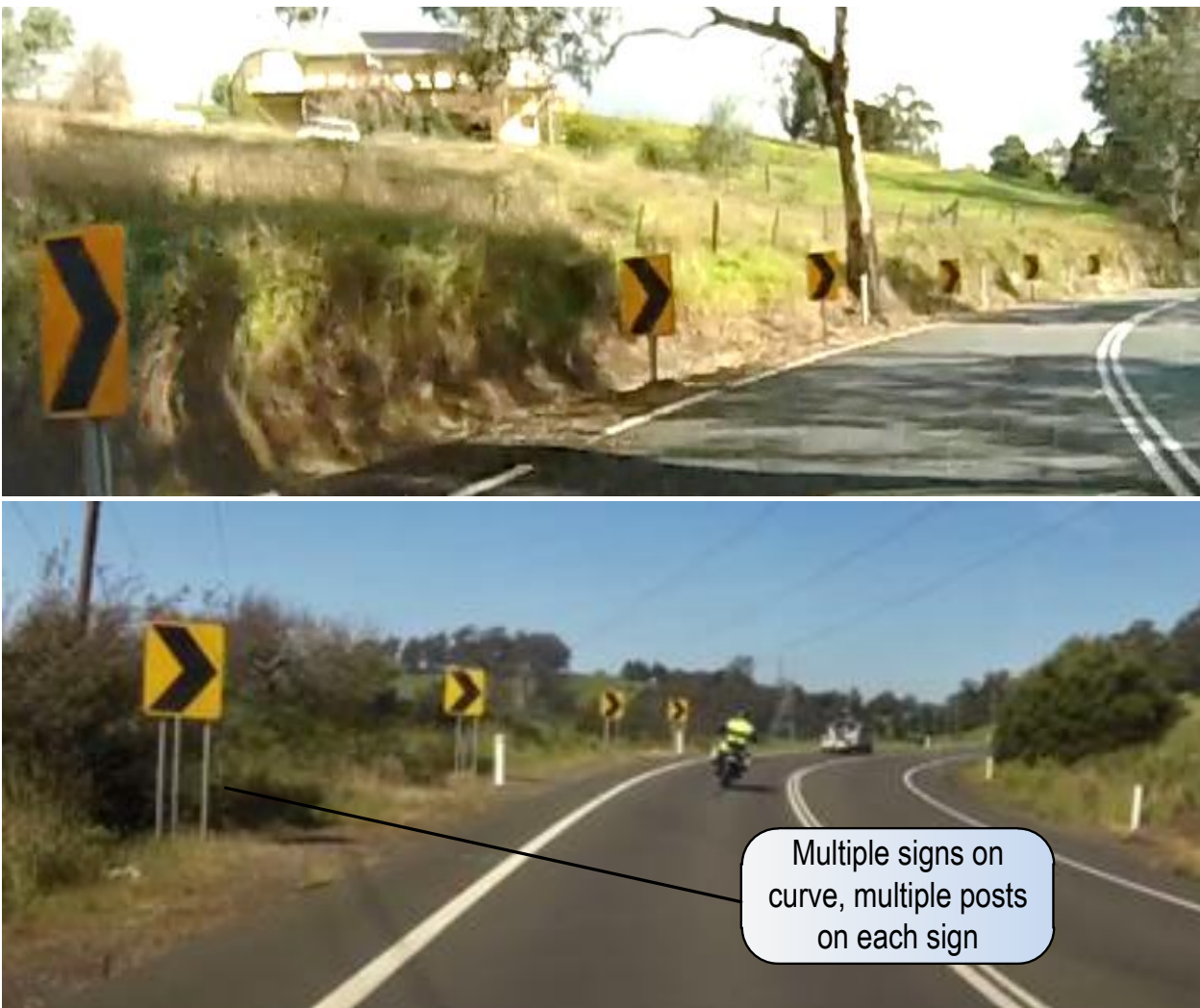
Figure 4.105: Multiple sign posts on the outside of a curve
