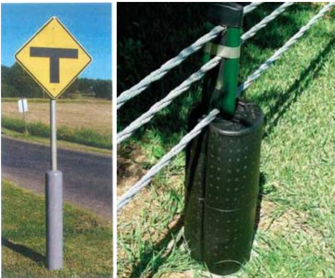
Figure 5.14: Sign post (a) and wire-rope barrier post (b) impact absorbing pads (see Section 1.4)
