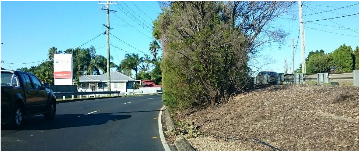
Figure 4.18: Restricted sight lines – right hand curve divided carriageway
