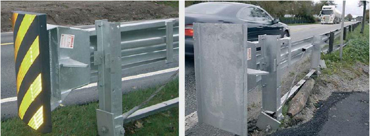
Figure 4.111: End terminal (ET2000) with and without cover
