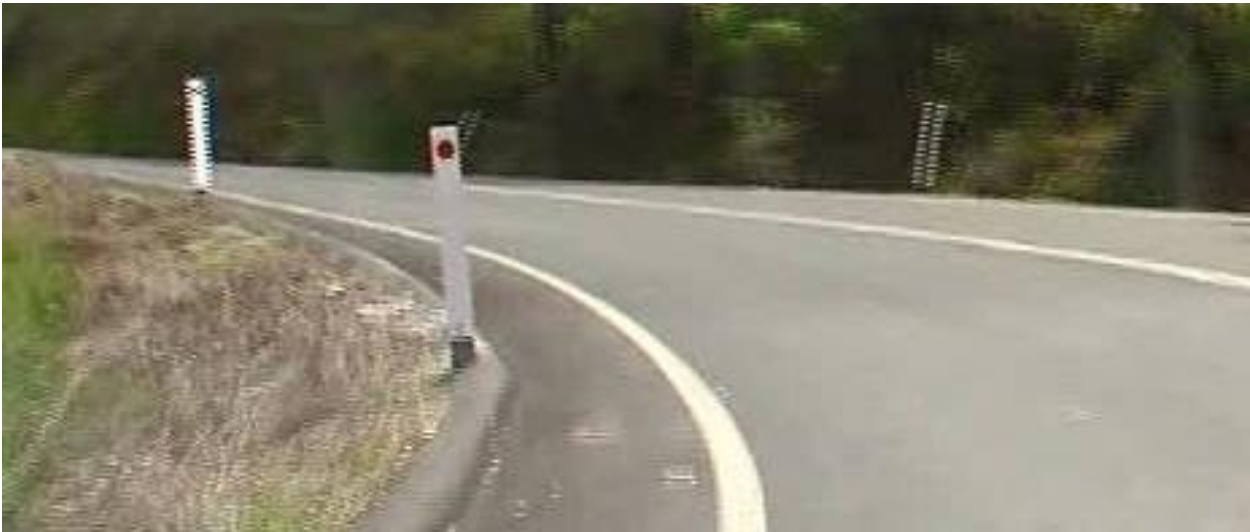
Figure 4.63: Cold mix kerbing, not conspicuous
