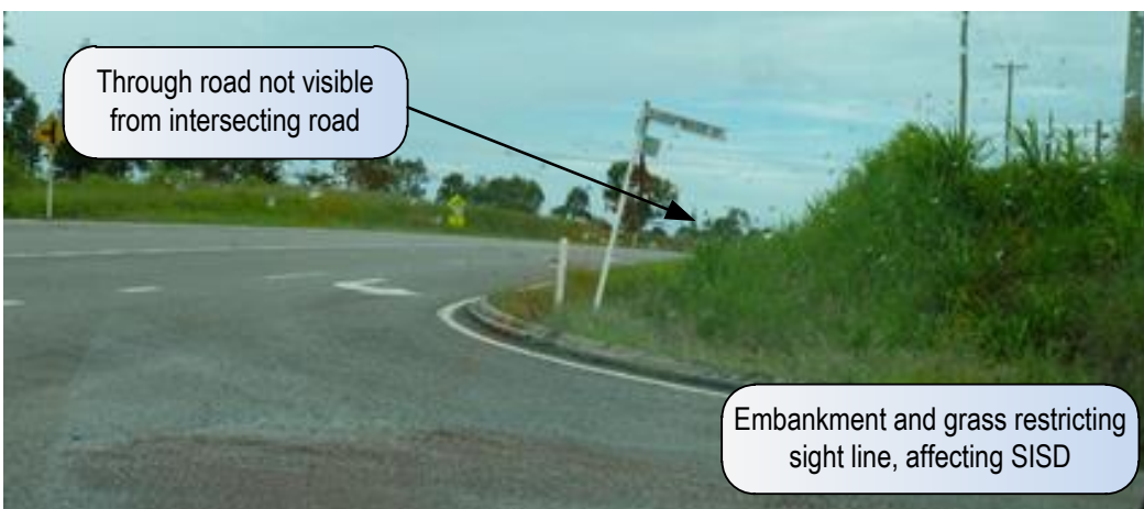
Figure 4.80: Rural – restricted safe intersection sight distance
