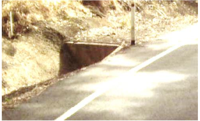
Figure 4.118: Culvert end wall and gully pit wall perpendicular to through road
