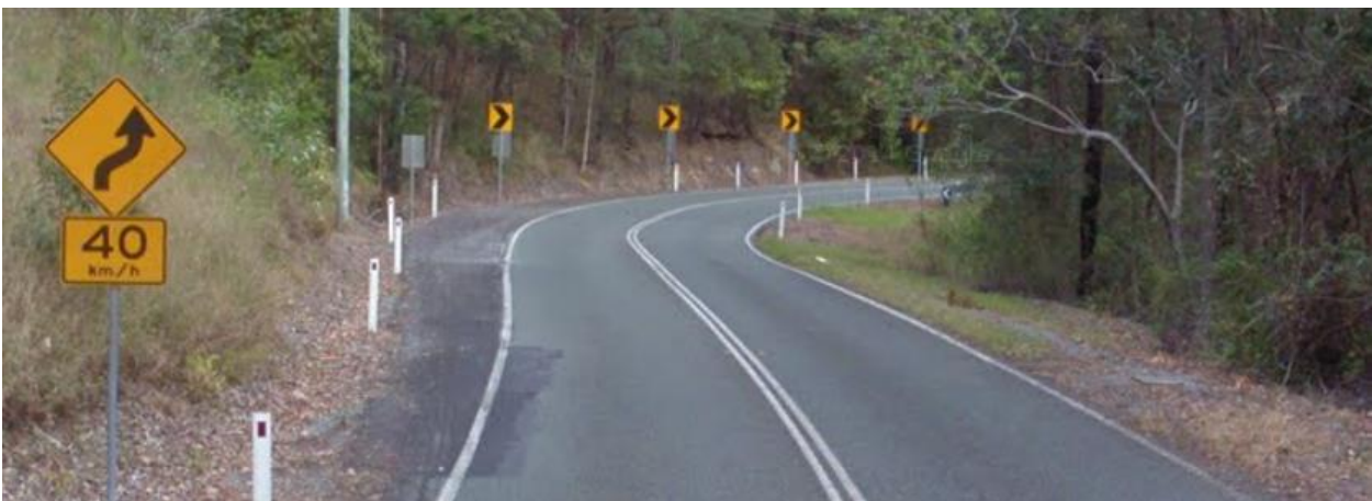
Figure 4.39: Curve warning sign and CAMs confirming direction of the first curve in this series of curves
