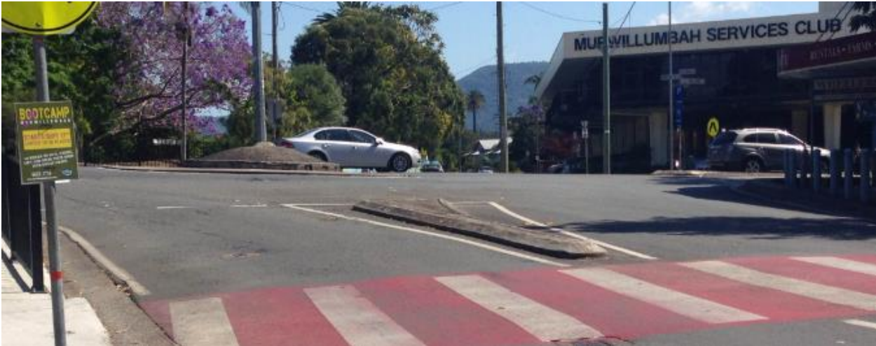
Figure 4.53: Pedestrian crossing pavement marking in braking zone
