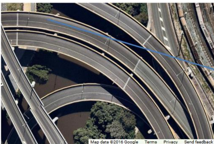
Figure 4.58: Multiple bridge joins on a curve with restricted sight lines
