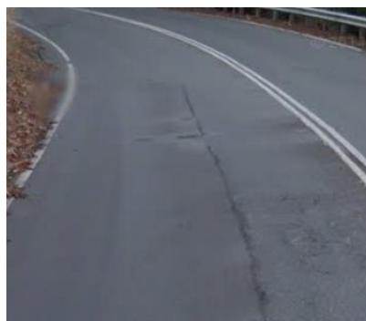
Pavement repair construction joint on curve
