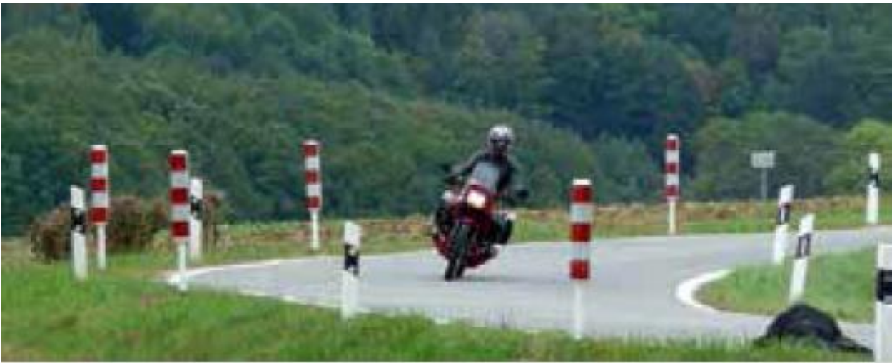
Figure 4.38: Flexible bollards do not indicate direction of the curve from the approach
