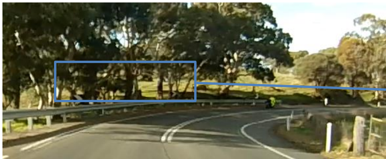
Figure 4.45: CAMs not conspicuous and hazard markers used
