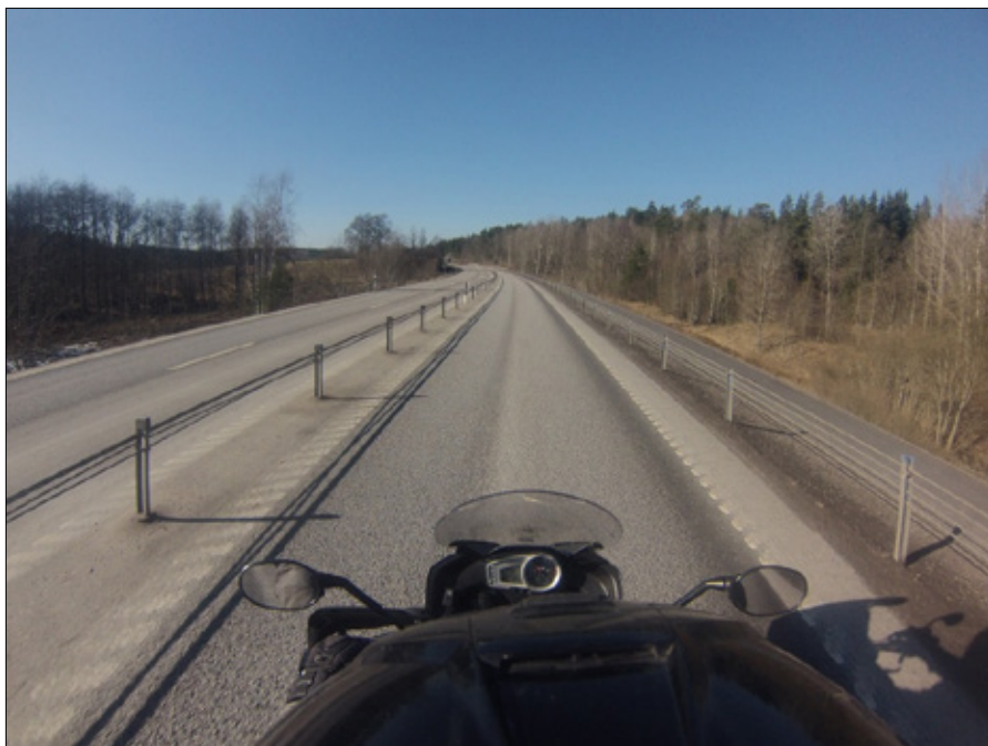
Picture 2. Cable barrier installation 2+1 in Sweden (Finspång-Norrköping).
