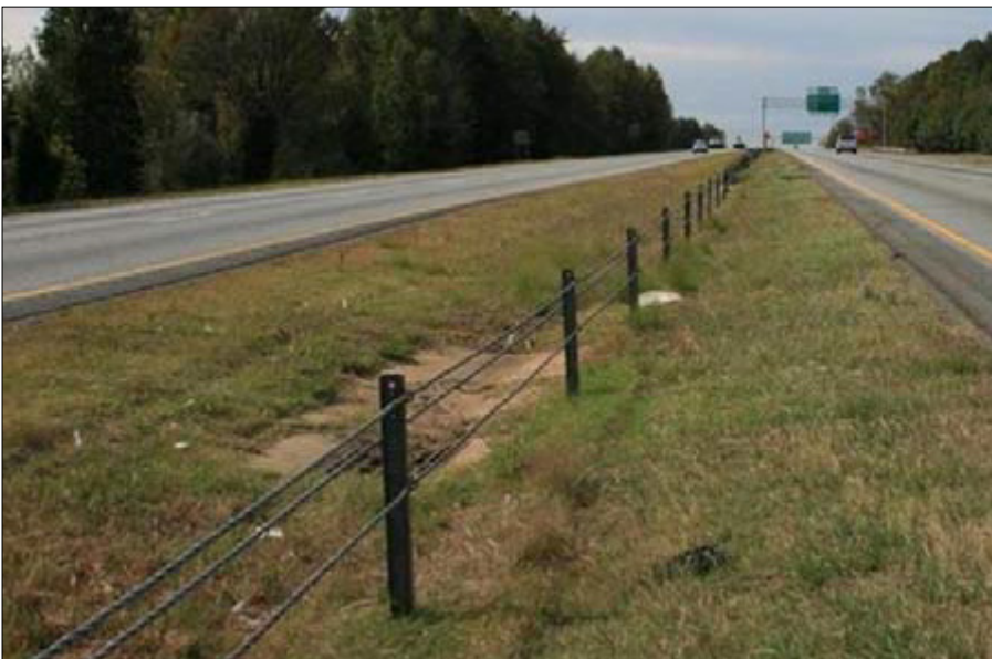
Picture 1. Median cable barrier installation in USA
