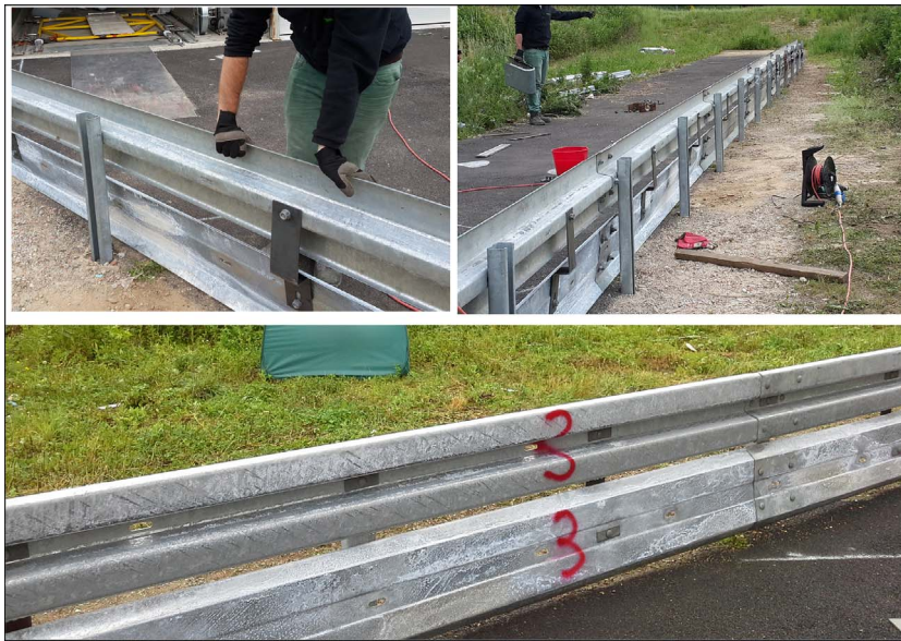
Fig. 16. Completed CMPS installation before crash testing.
