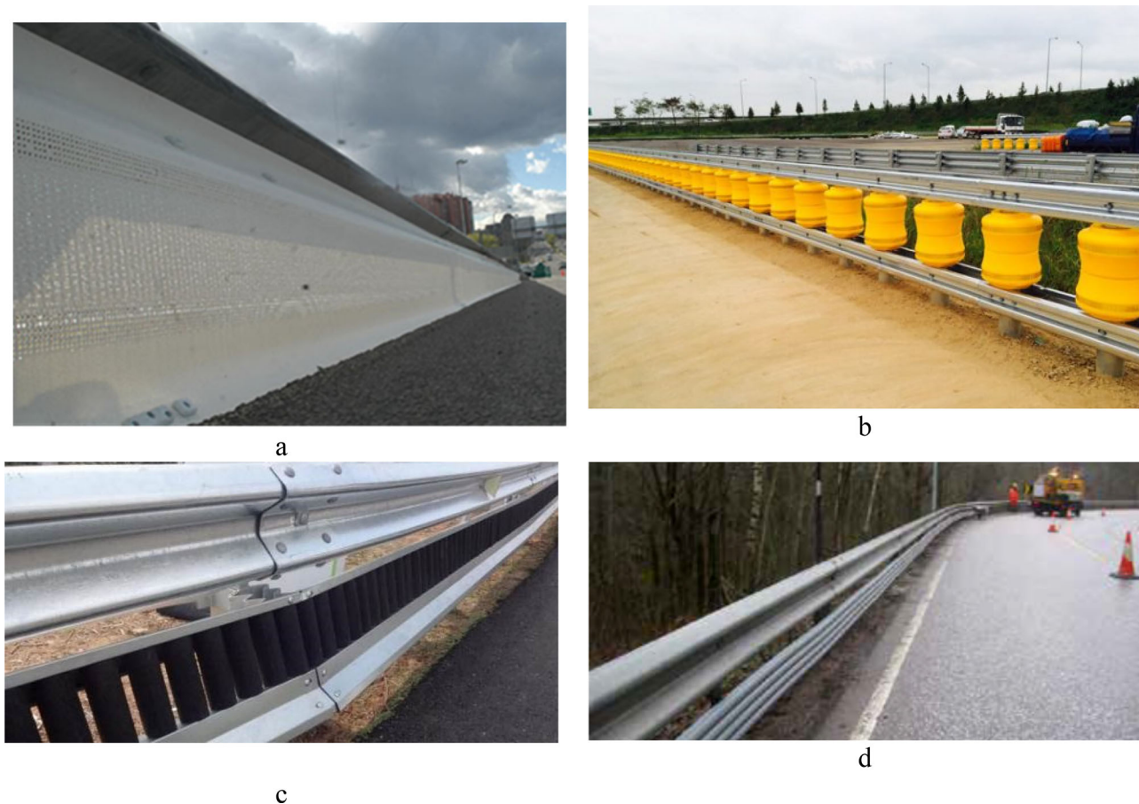
Figure 3. Continuous MPS made from materials other than steel: a) Basic fabric [7], Shindo Safety polyethylene roller [10]; c) Segurvital recycled rubber [11], Swedish polyethylene tubular subrail [12].
